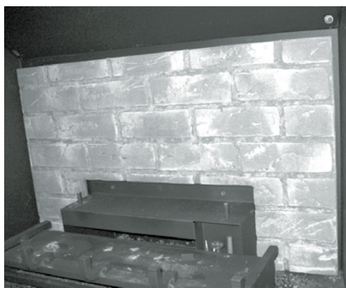
Back Panel Installed
