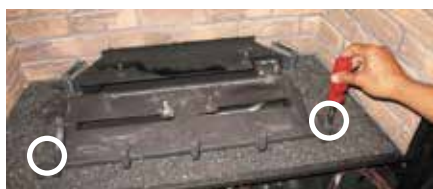
Diagram 1: Remove the left and right screws.
