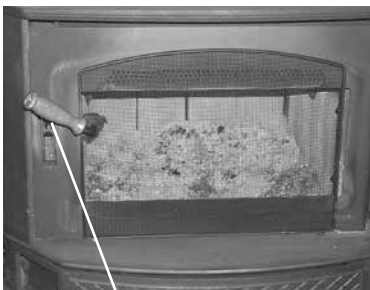
Handle at 10 o'clock position.
