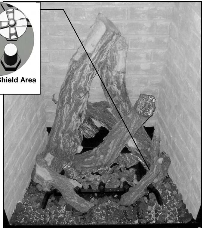
Step 6: Add lava rock to the bottom of the burner pan. Add glowing embers to the top of the ember plates and front burner tube. Sprinkle vermiculite over the lava rock. Do not place any media within Pilot Shield Area (see above).
