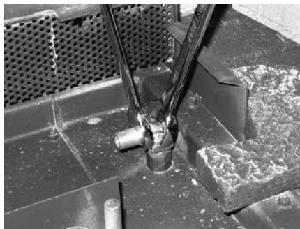
Burner Orifice Removal
