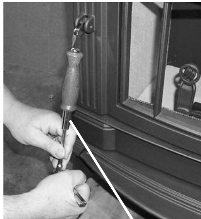
Secure using 7/16" socket wrench.
