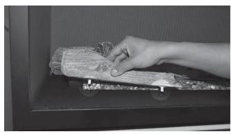
4. Place the right rear log as indicated. Pivot tail end to just cover small hole located in platform.
