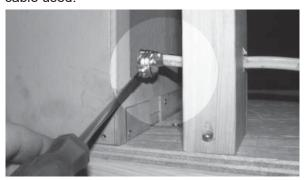
8. Tighten cable clamp on outside of fireplace casing and secure and excess wire to framing.
