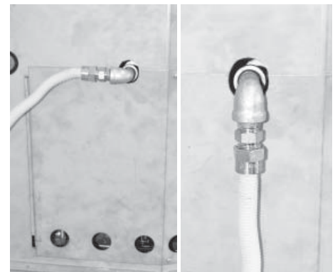
Flex connector redirected using two elbows.
