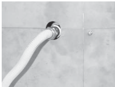
Flex connector redirected using one elbow.
