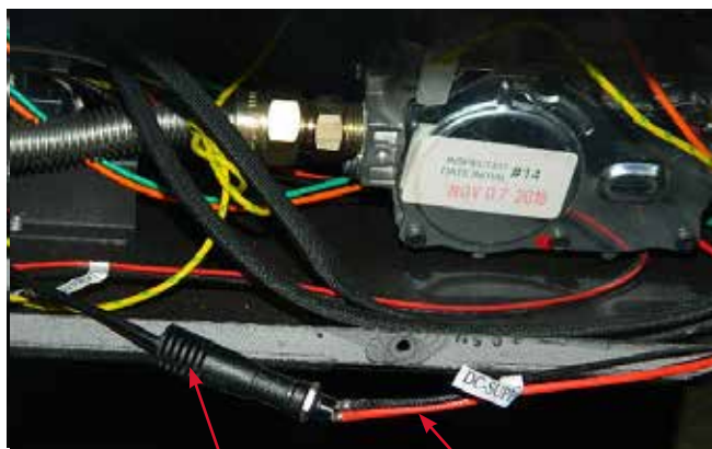
DC supply wire from wiring harness
