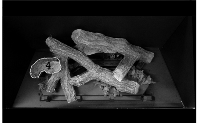
STEP 4: Place Log #4 into place as shown. Do Not place directly over top of the multiple porting area on the left side.
