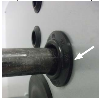
FIGURE 27 - FURNACE GAS PIPE CONNECTIONS (NOTE RUBBER GROMMET)
