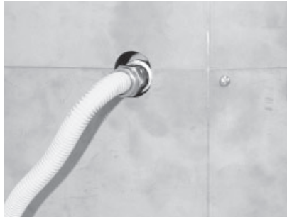
Flex connector redirected using one elbow.
