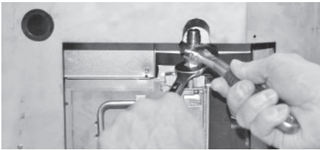
Flex connector redirected using one elbow.
