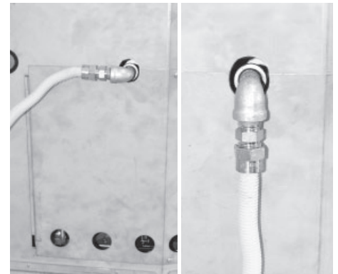
Flex connector redirected using two elbows.
