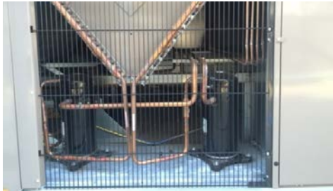
Compressor access for “Magnum” style units
