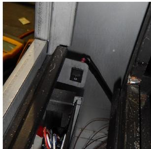
8. Place Fan wire on leftside firebox floor with adhesive wire pad. For fan Install instructions see **Optional fan kit Install/Replace instructions**
