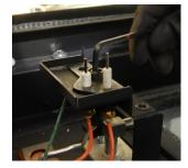
Figure 13.e Removing the pilot hood, orifice
