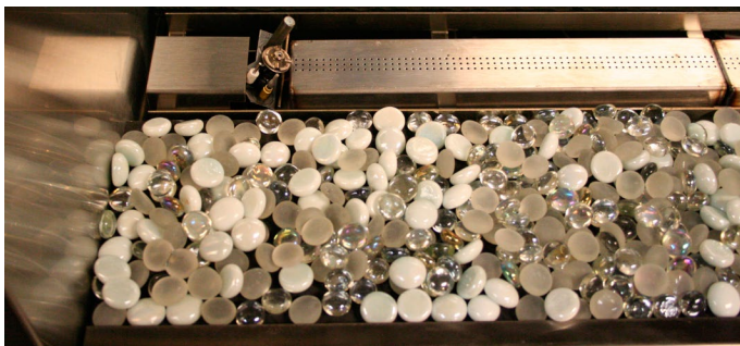
Figure 12. Installation of glass beads . Note: Ensure the beads do not cover the burners or pilot.
