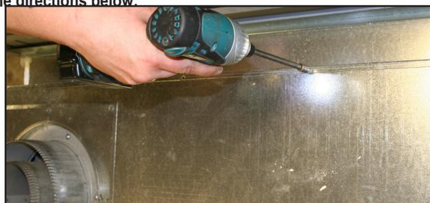
Figure 7. Remove screws from top of the unit
