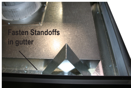
Figure 6. Installing the H*38PR* standoffs.
