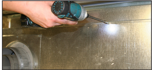
Figure 7. Remove screws from top of the unit
