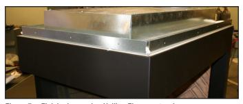
Figure 7c. Finished removing Nailing Flange extension.
