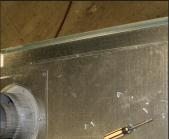
Figure 7b. Remove the nailing flange extension from the unit. Reinstall shell and insulation. Screw shell in place.
