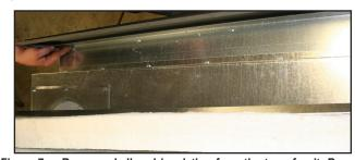
Figure 7a. Remove shell and insulation from the top of unit. Remove screws from outer edge.
