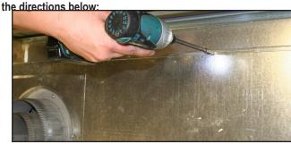
Figure 7. Remove screws from top of the unit
