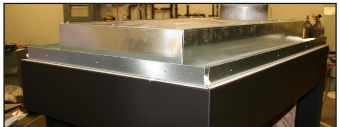
Figure 7c. Finished removing Nailing Flange extension.
