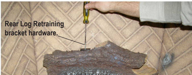
Figure 31b. Fastening Retaining bracket to Rear Log.
