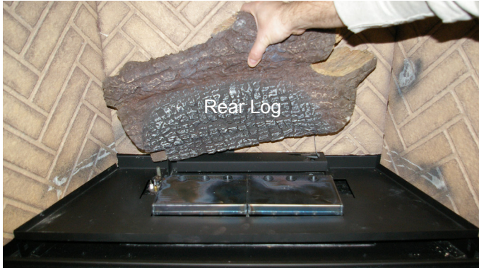
Figure 31. Rear log alignment.
