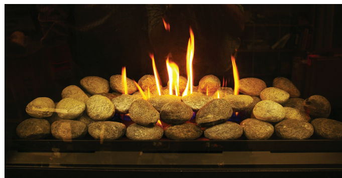
Figure 30h. Completed Placement. Note: You may have to adjust the Faux rocks to produce a pleasing flame pattern and reduce sooting. (as shown)
