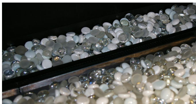
Figure 28. Completed firestone installation. Second Gen burner shown.
