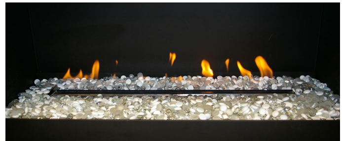
Figure 24a. Operating gas fireplace with firestones surrounding burner tray. Second Gen Burner Shown
