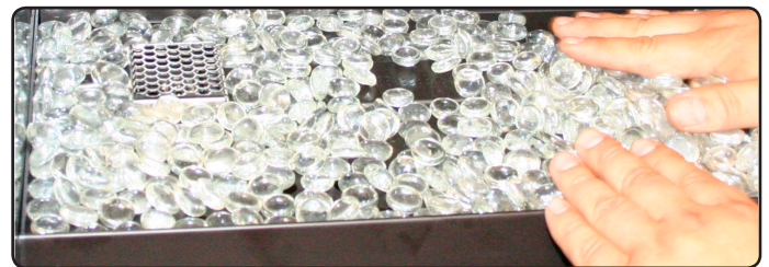
Figure 24. spreading out firestones
