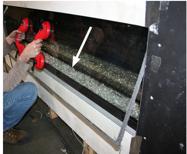
Figure 2 Sec.8 Window Removal (using glass lifting tools).
