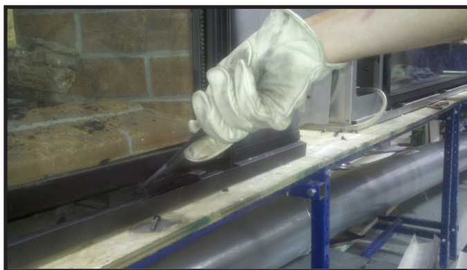
Figure 11.3. Inserting Glass Clip Tool
