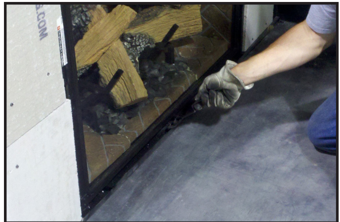
Figure 11.8. Securing Bottom Glass Clips
