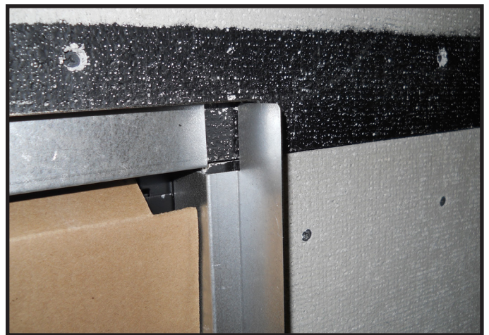
Figure 10.5 Finishing Template Bends
