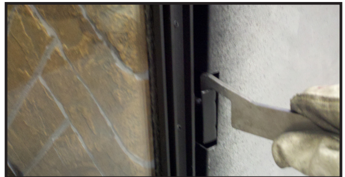
Figure 11.7. Securing Side Glass Clips
