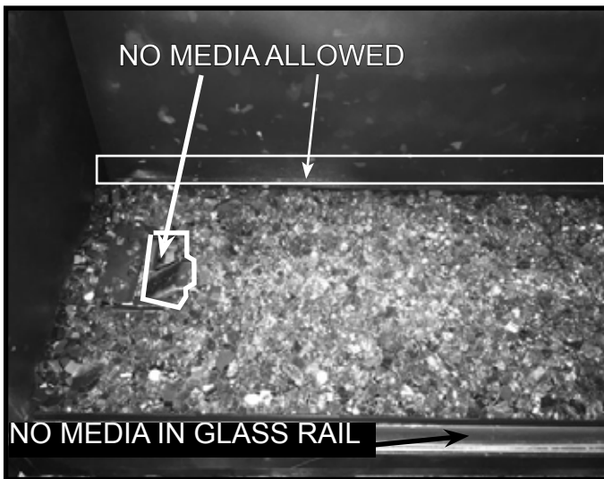
Figure 6. Media Installed
