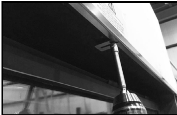
Figure 10.5. Install Trim Ring
