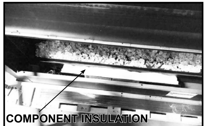
Figure 11.3 Component Insulation Location
