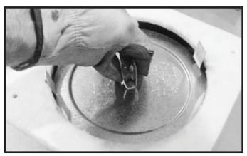
**Figure 6.4** Fold the center parts of the retaining band up and use to remove the vent cap.
