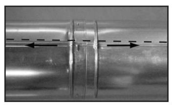
Figure 7.11 Align and Disassemble Vent Sections
