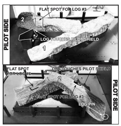
Figure 4. Log #2 Installed - View From Both Sides
