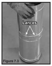
**Note:** Make sure that the seams are not aligned to prevent unintentional disconnection.
