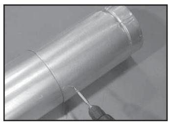
Figure 7.7 Screws into Slip Section
