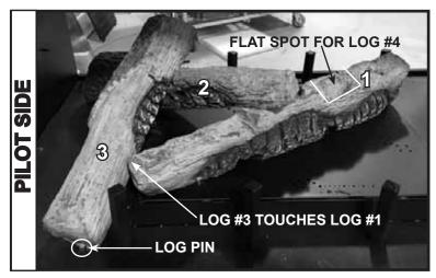
Figure 5. Log #3 Installed
