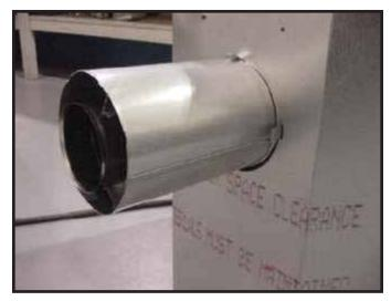
**Figure 6.9** Attach the first vent section (it will snap into place). Slide the vent gasket onto the vent section and then, up against the appliance. Secure the vent gasket to the appliance with two self-tapping screws found in the manual bag. Note: The vent gasket can found in the manual bag.
