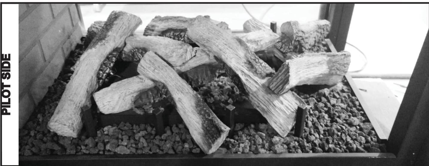
Figure 14. Log Set Installed
