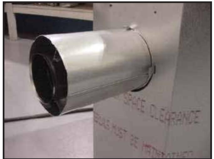
**Figure 6.9** Attach the first vent section (it will snap into place). Slide the vent gasket onto the vent section and then, up against the appliance. Secure the vent gasket to the appliance with two self-tapping screws found in the manual bag. Note: The vent gasket can found in the manual bag.
