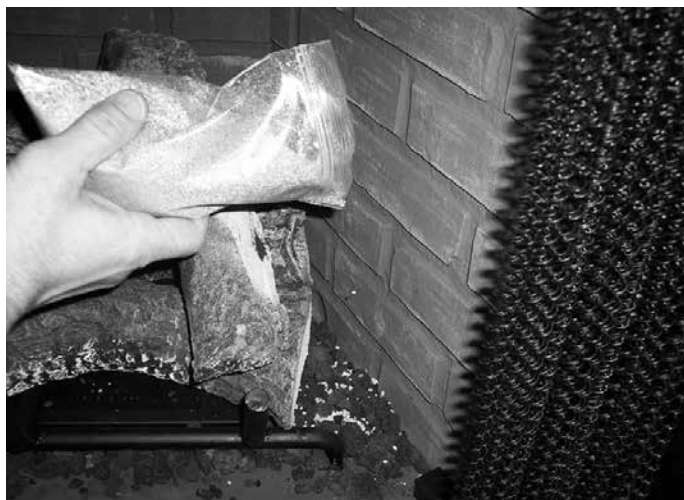
Figure 14.22 Placement of Vermiculite
