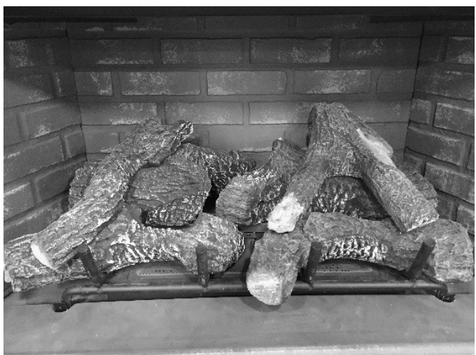
Figure 14.20 Final Log Placement
