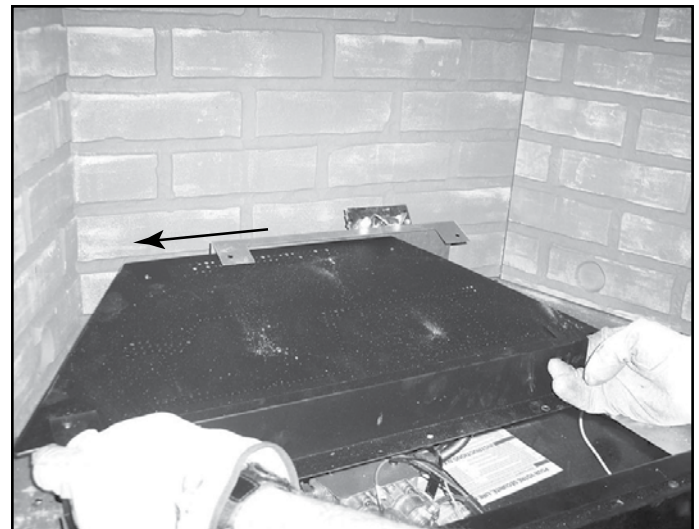
Figure 14.30 Side Burner Assembly to Left
