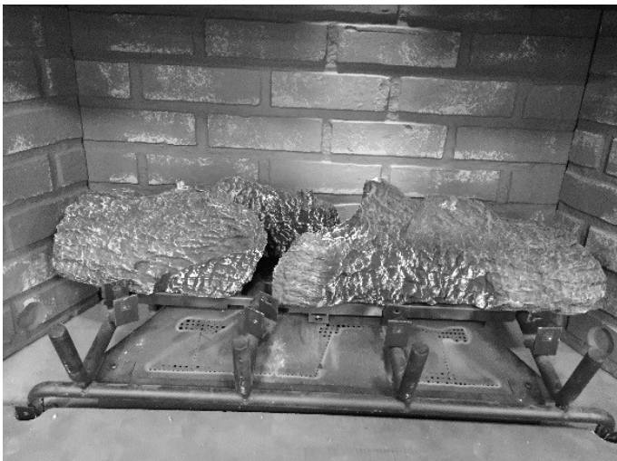
Figure 14.8 Left and Right Rear Log Placement
