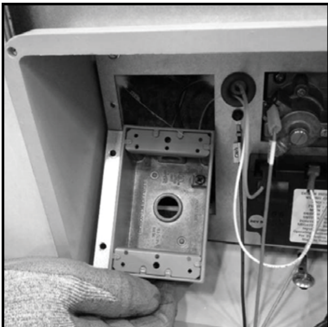
Figure 5.6 Place & Fasten Junction Box
