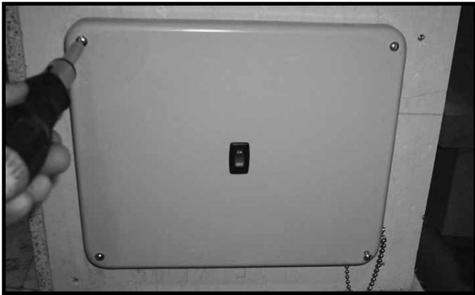
Figure 5.1 Remove Control Cover
