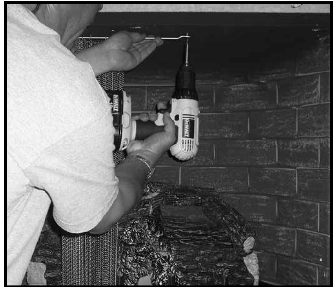
Figure 8.17 Fasten Screen Rod to Firebox Top
