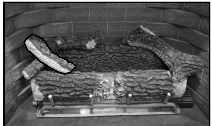
Figure 8.10 Place Top Log on Left Side
