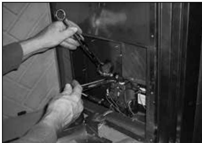
Figure 12.6 Turn off Gas Valve
