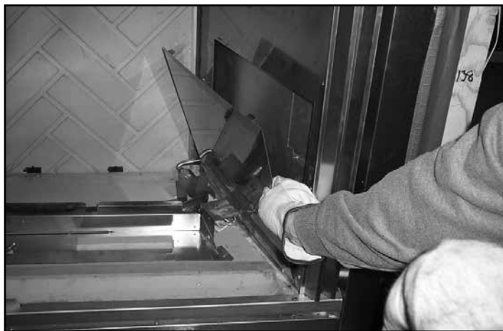
Figure 12.4 Remove Valve Access Panel
