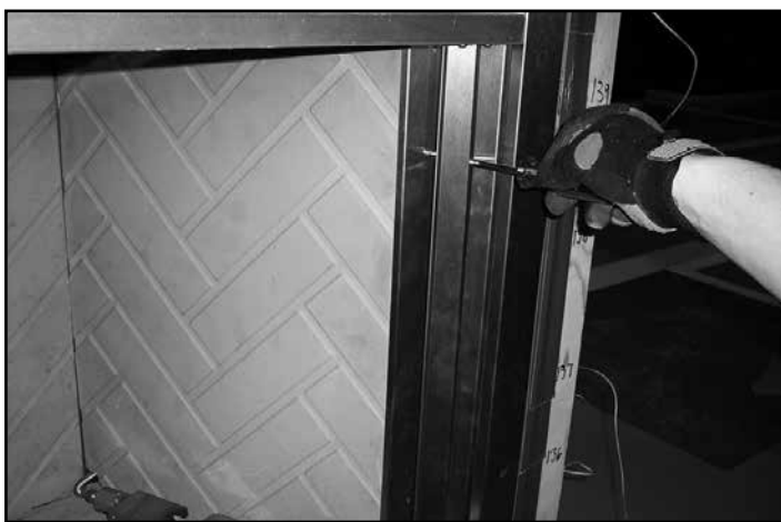
Figure 12.3 Loosen Refractory Retaining Strip
