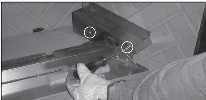
Figure 6.2 Remove Pilot Shield
