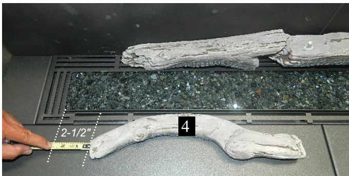
Log 4 to edge of burner
