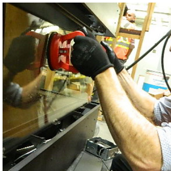
Handle glass with supplied vacuum clamps
