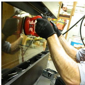
Handle glass with supplied vacuum clamps
