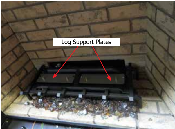
Diagram 6—Log support plates installed
