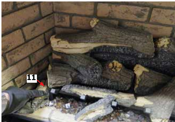
Diagram 17—Install Log 11
