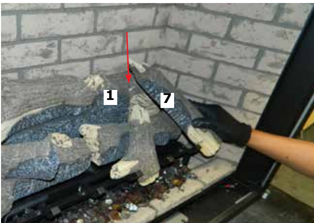
Diagram 13—Install Log 7
