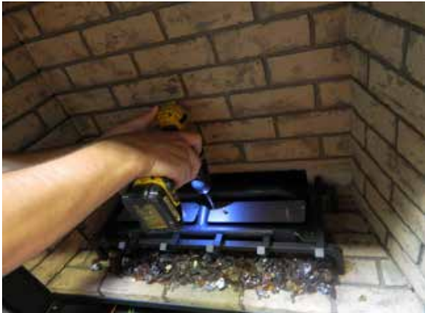
Diagram 5—Install Log support plates
