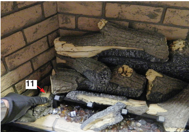
Diagram 18—Install Log 11
