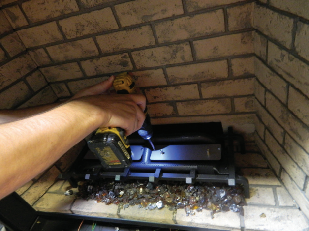
Diagram 5—Install Log support plates
