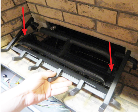
Diagram 1: Remove the left and right screws.
