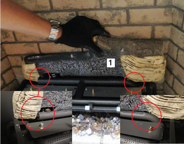
Diagram 7—Log 1 installation
