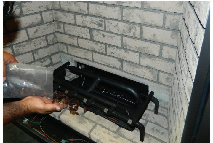
Diagram 3—Install Glass
