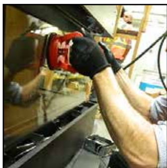
Handle glass with supplied vacuum clamps
