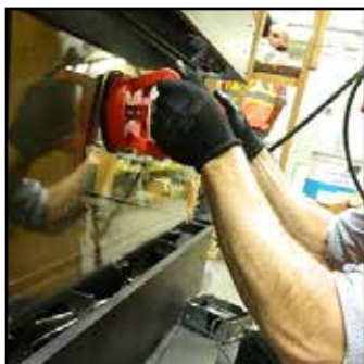
Handle glass with supplied vacuum clamps
