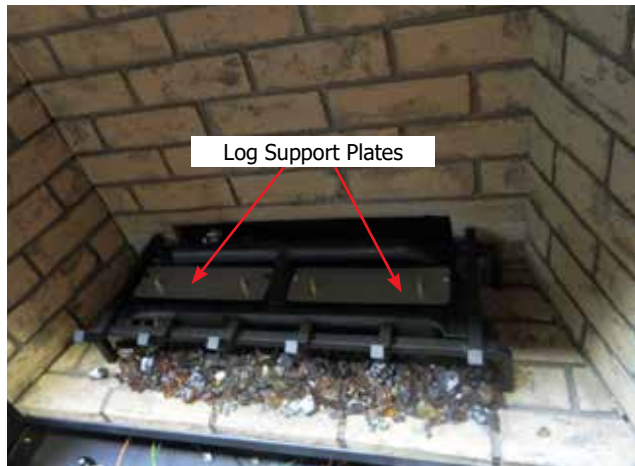
Diagram 6—Log support plates installed
