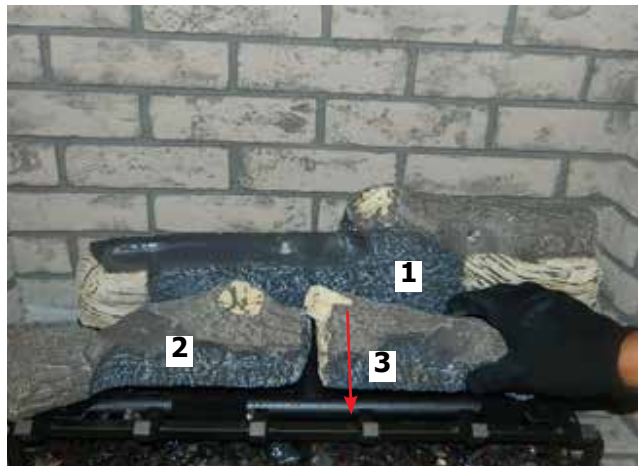
Diagram 9—Install Log 3
