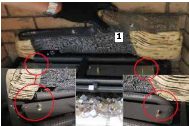
Diagram 7—Log 1 installation
