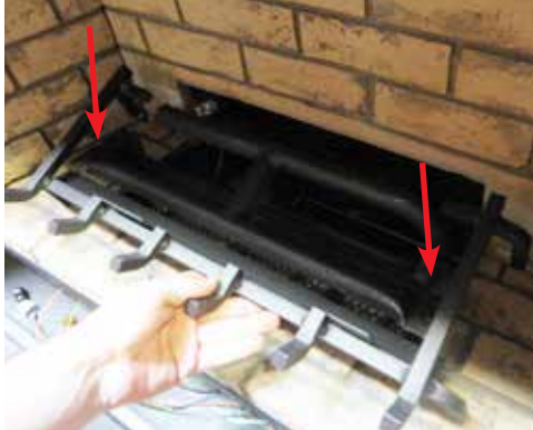
Diagram 1: Remove the left and right screws.
