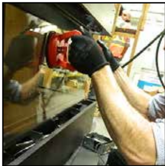
Handle glass with supplied vacuum clamps
