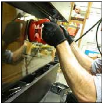
Handle glass with supplied vacuum clamps
